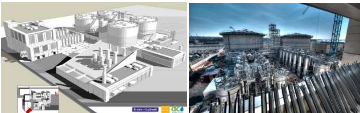
(left) 3D view of Cambi THP and digestion design and (right) a view of Cambi THP and digesters from dewatering house on the corner
