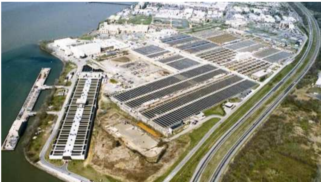
Fig. 4. A bird view of existing Blue Plains AWTP
